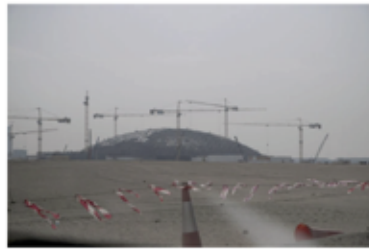
Louvre Museum Construction, Abu Dhabi, March 2015.
